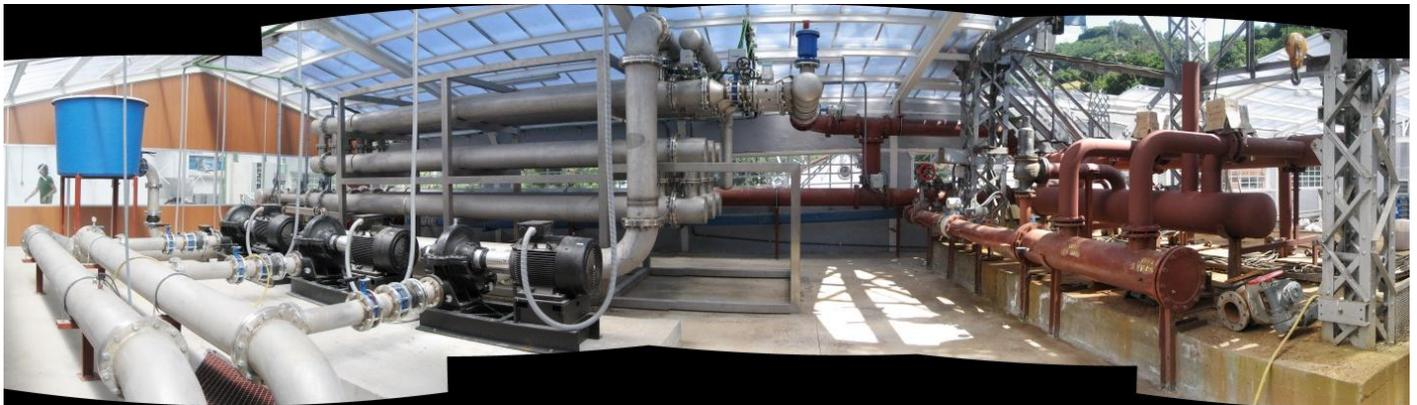
Figure 18. Heat exchanger in Barredo Shaft
