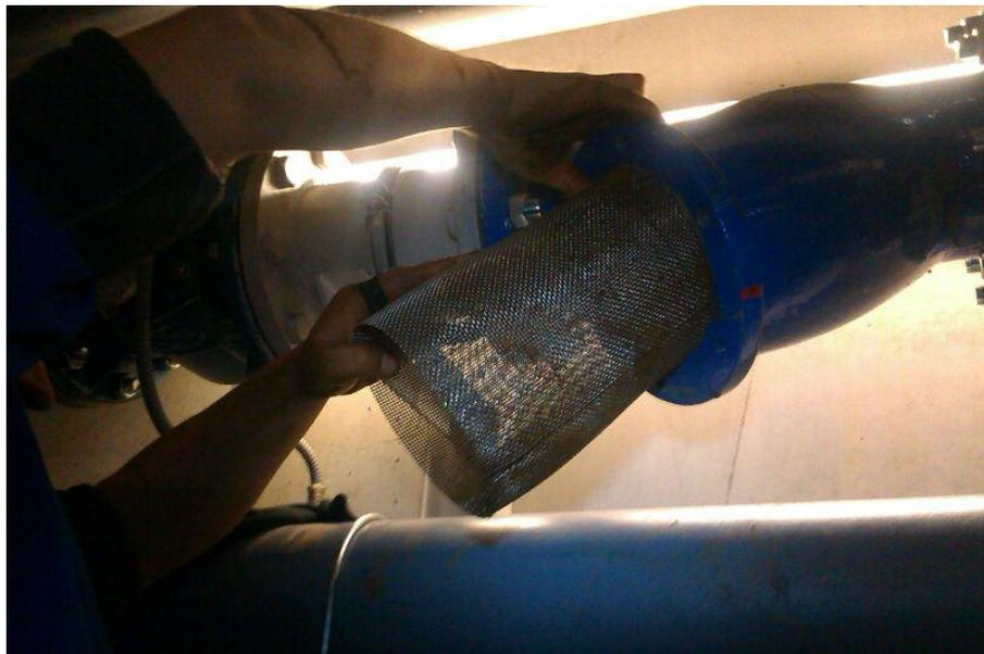
**Figure 17. Filter after cleaning.**
