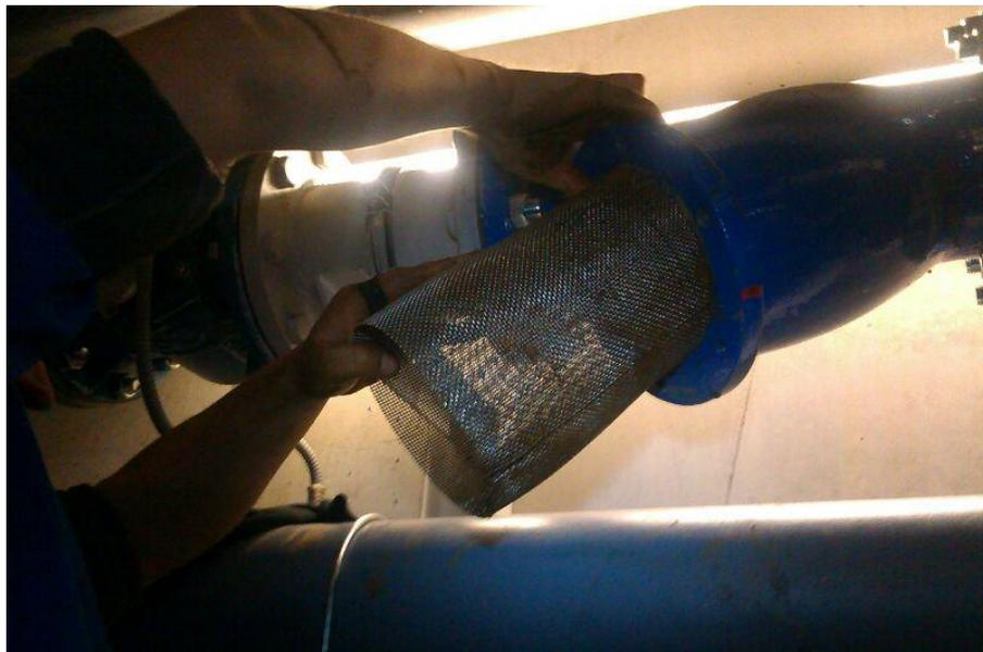
**Figure 17. Filter after cleaning.**
