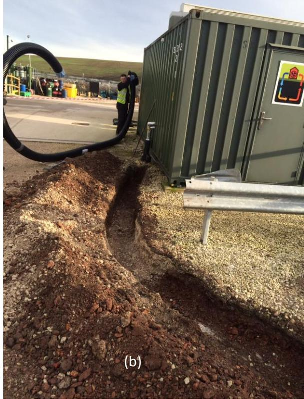
**Figure 20: Pipes being laid to convey hot water from (a) GSHP container (b) Engine**
