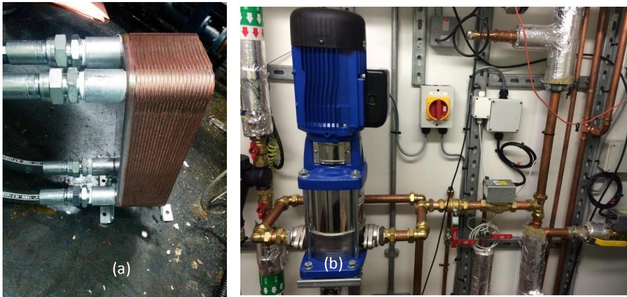
**Figure 19: (a) Plate heat exchanger on the engine side to transfer and recovery heat. (b) Circulation pump to circulate heat to the engine.**
