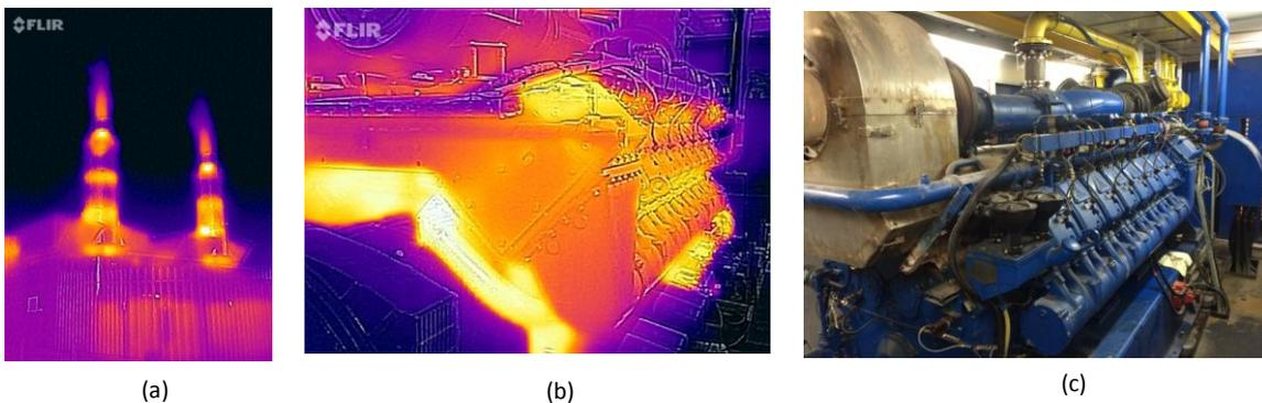
**Figure 18: (a) The thermal image of the engine in operation mode. (b) The thermal image of the engine in standby mode. (c) Normal image of the engine.**
