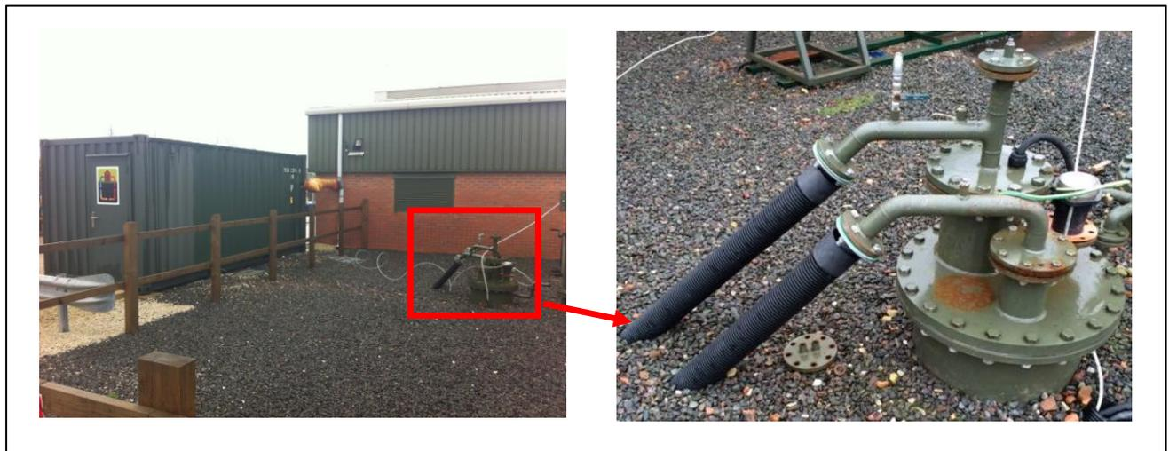
Figure 5: Mine water flow and return pipe.
