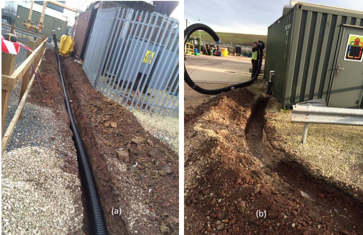
**Figure 20: Pipes being laid to convey hot water from (a) GSHP container (b) Engine**
