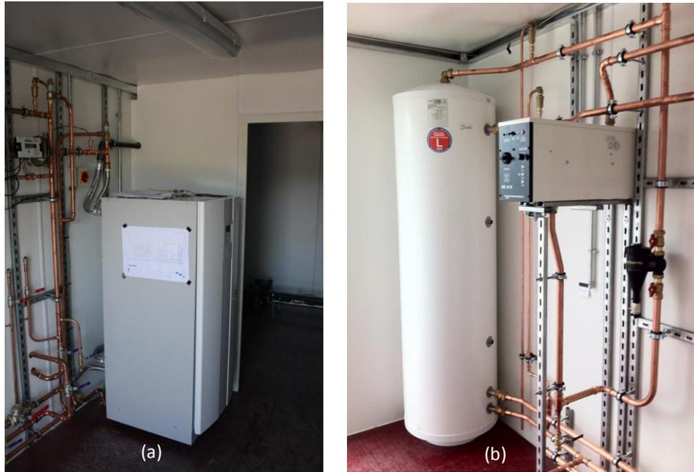
**Figure 8: (a) Heat pump. (b) Buffer tank.**
