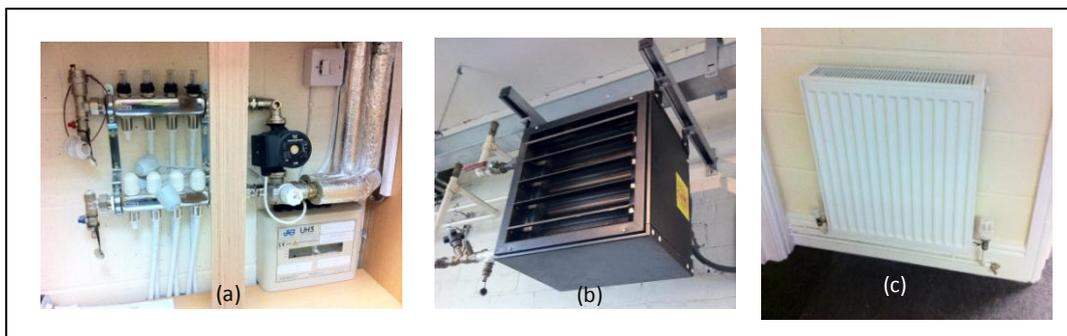
**Figure 10: The Emitter systems used to dissipate the heat**
