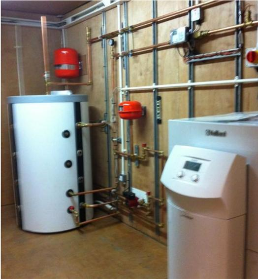
Figure 6: Heat pump and the Buffer tank
