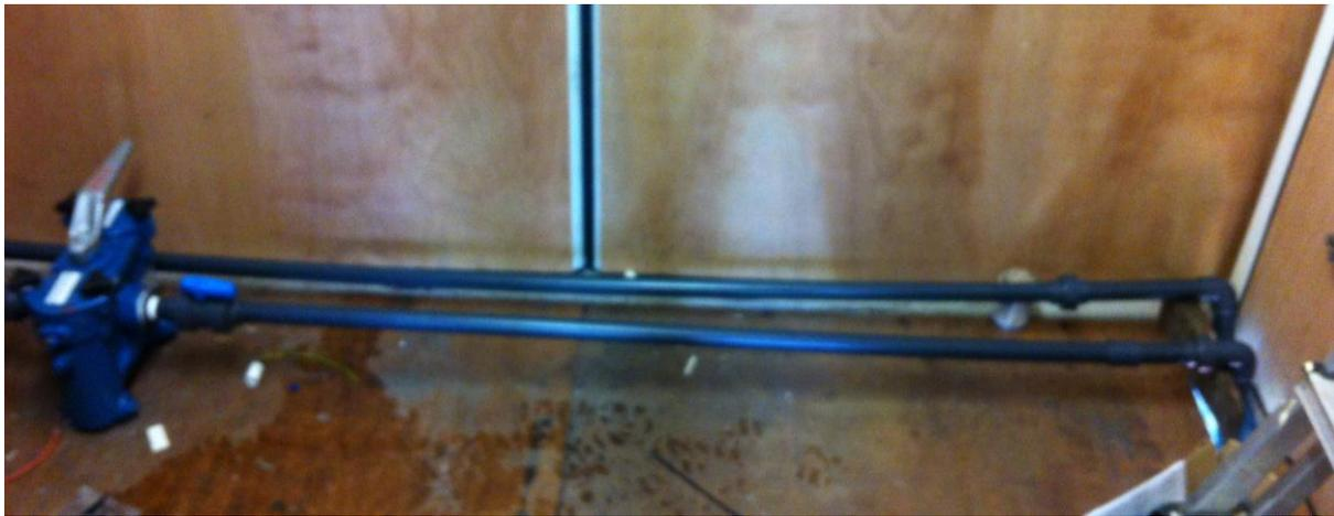
Figure 14: A duplex filter to remove ochre and other suspended particles
