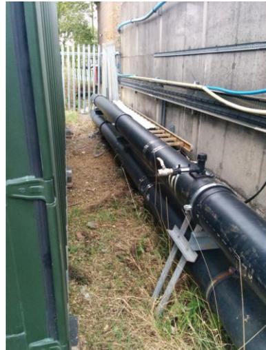
Figure 9: mine water being tapped for the pilot plant from the main line
