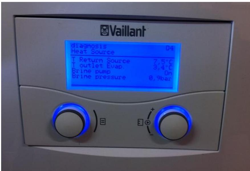
Figure 11: Heat pump displaying the brines temperatures
