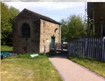
Inman shaft building
