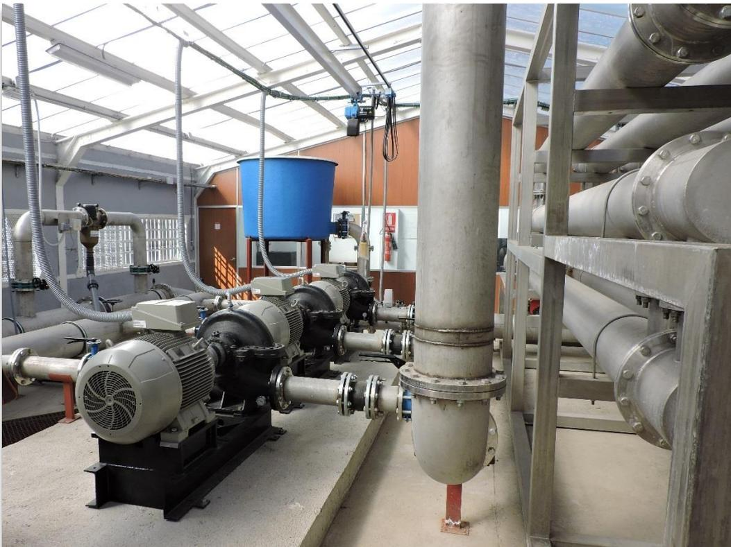
**Figure 6.17. Shell-and-tube heat exchangers (right) and circulation pumps on secondary circuit to hospital, Barredo shaft-top building.** Photo by © David Banks
