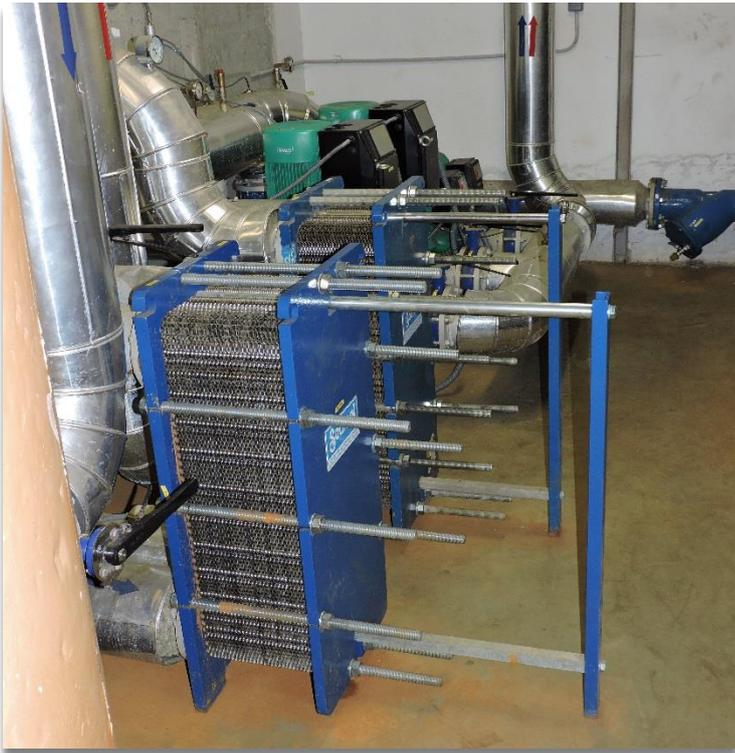
**Figure 6.5. Mine water to secondary circuit plate heat exchangers. Mieres university building. Photo by © David Banks**
