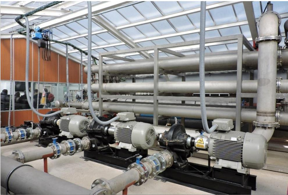
**Figure 6.15. Shell-and-tube heat exchangers between mine water and secondary circuit (with circulation pumps) to hospital, Barredo shaft-top building.** Photo by © David Banks
