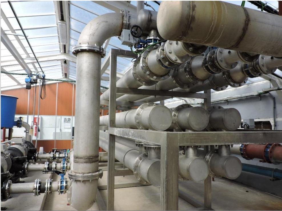
**Figure 6.16. Shell-and-tube heat exchangers between mine water and secondary circuit to hospital, Barredo shaft-top building.** Photo by © David Banks
